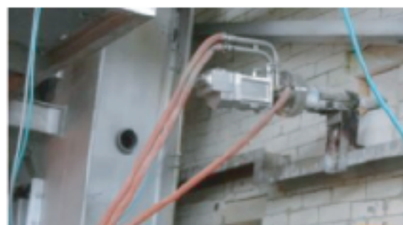
▲ 24/7 Operation and Remote Process Monitoring
